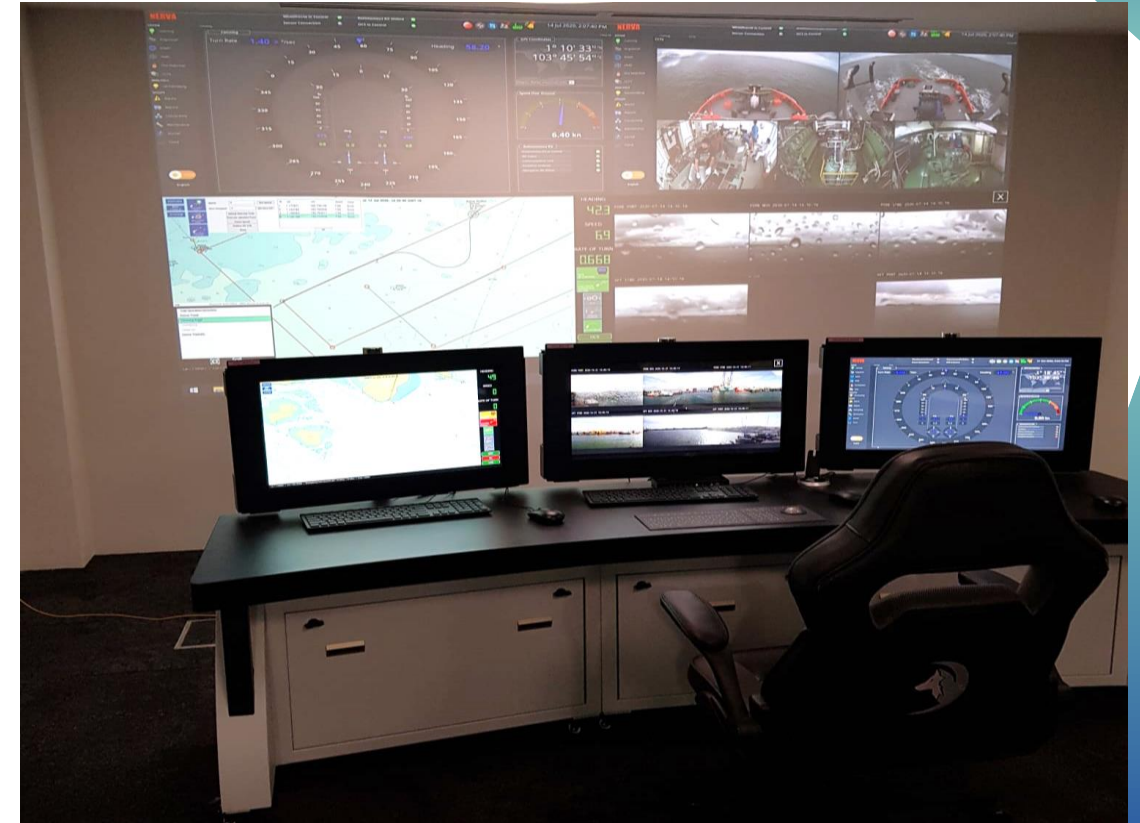
Set-up of shore command centre
